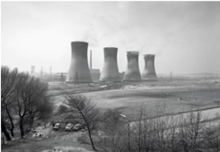
Agercroft Power Station, Salford, 1983
